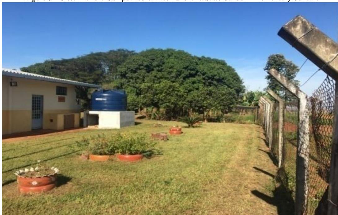
Figure 3 - Cistern of the Campo Padre Antônio Vieira State School - Elementary School.
